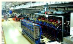
Inside view of the IR-FEL facility at RRCAT
