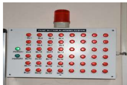
Fig. E.8.3: Indicator panel with audio/visual alarming
