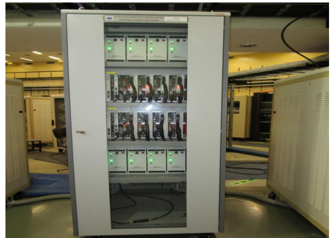
Fig. A.3.1: Equipment controllers in a control cabinet.
