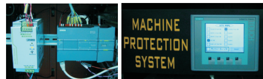
Fig. A.12.4: PLC based Machine Protection System.
