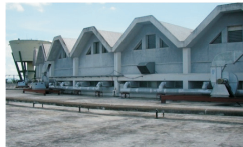
Fig. I.3.3: Two zones of smoke exhaust system installed on the roof of Indus Accelerator Complex.
