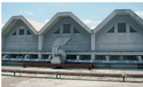
Fig. I.3.1: A portion of the smoke exhaust system covering three sectors of a zone with a direct driven blower.
