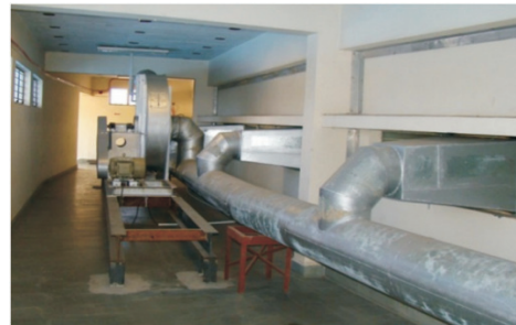
Fig. I.3.2: The smoke exhaust system with a belt-driven blower catering to MPS area of Indus-2 accelerator.
