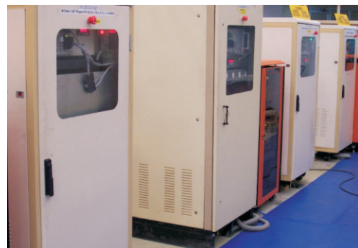
Fig. A.1.2: Photograph of the new power converters installed and operational in Indus-2.
