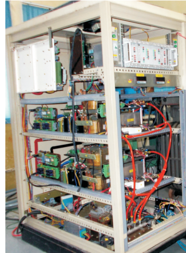
Fig. A.1.1: Photograph showing assembly details of a cabinet housing two power converters.
