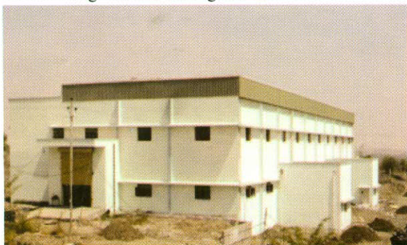
Fig. I.1.2: Roadside view of the H - ion lab buildings
