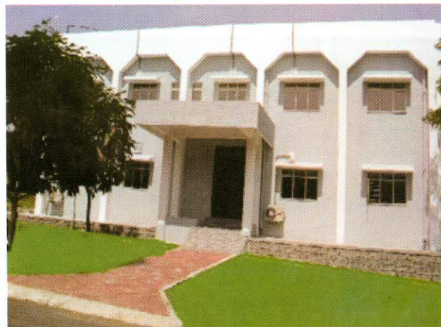
Fig. I.1.3: Front view of the Communication building
