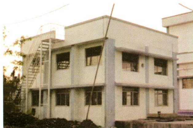
Fig. I.1.4: A view of the LCW Plant building
