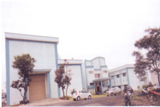
Figure I.4.2: View of UHV –MFL Building
