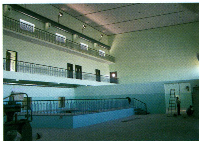
Figure I.6.2: View of high bay to house test stand for cavity
