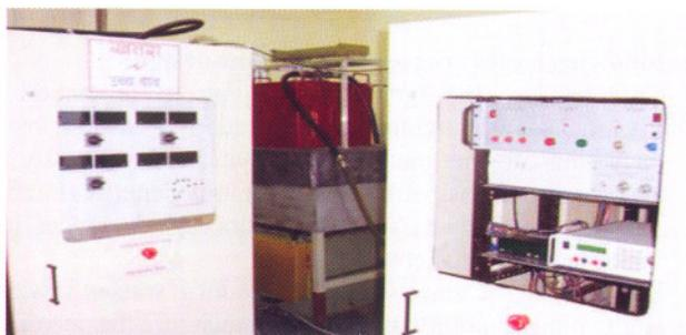
Fig. T.1.11: Microwave system installed in equipment room of 10 MeV LINAC.
