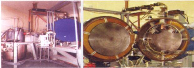
Fig T.1.7: 5 MW Microwave system and microwave cavity installed in 20 MeV Microtron at RRCAT.
