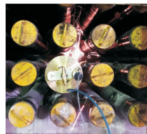
Fig. L.2.1: In-situ laser cutting of bellow lip weld joint at KAPS-2 reactor
