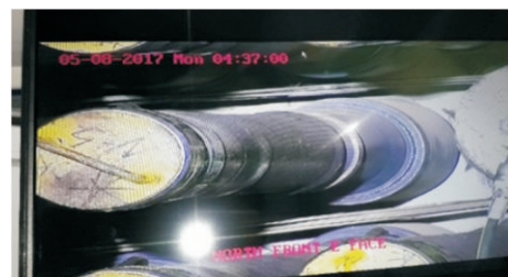
Fig. L.2.2: Laser cut and separated bellow lip weld joint for removal of coolant channel
